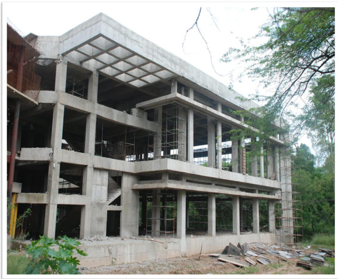
Auditorium still in steel and cement heading for completion
