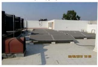
ii. 25 kWp SPV Power Plant at the New Block (Arbitration Centre), High Court Extension, Sector 17, Chandigarh, Cost of the plant is ₹ 20.66 Lakh and the Expected Power Generation on A.C. Side: Minimum 32,500 kWh (units) peryear.
