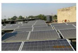
iii 25 kWp SPV Power Plant at the Old Block of High Court Extension, Sector 17, Chandigarh, Cost of the plant is ₹ 20.66 and the Expected Power Generation on A.C. Side: Minimum 32,500 kWh (units) per year.
